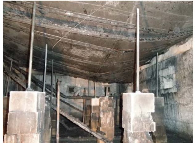
Figure 70. Exposed side from North end
