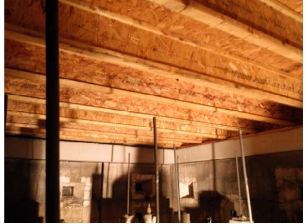
Figure 50. Pre-test exposed side
