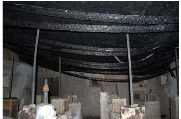
Figure 34. Exposed side from North end
