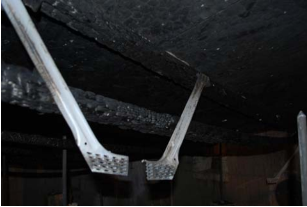
Figure 35. Joist with web disconnected
