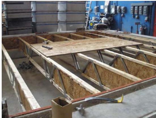
Figure 7 - Engineered Wood and Metal Hybrid Trusses
