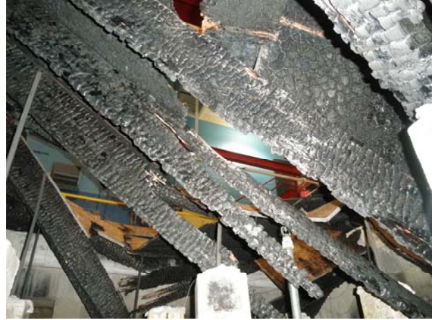
Figure 82. Exposed side from North end
