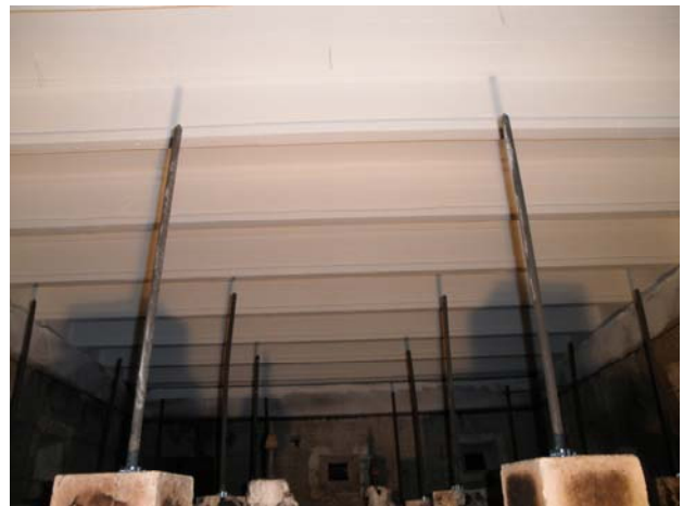
Figure 38. Pre-test exposed side
