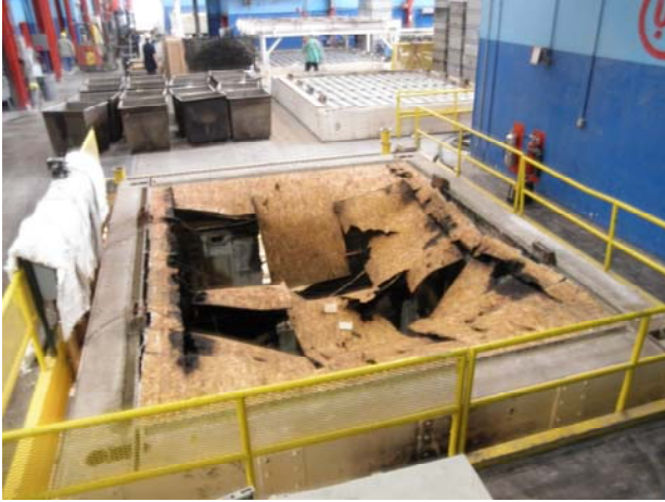
Figure 81. Unexposed side after collapse
