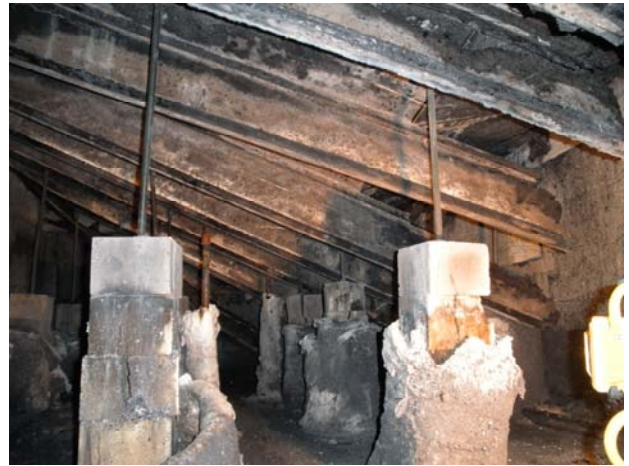
Figure 46. Exposed side from North end
