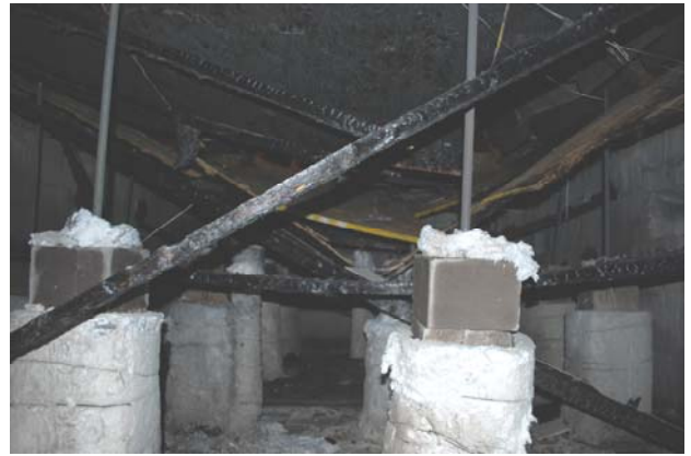
Figure 58. Exposed side from North end
