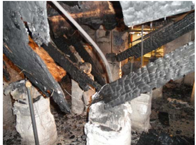
Figure 94. Exposed side from North end
