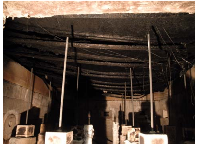
Figure 22. Exposed side from North end
