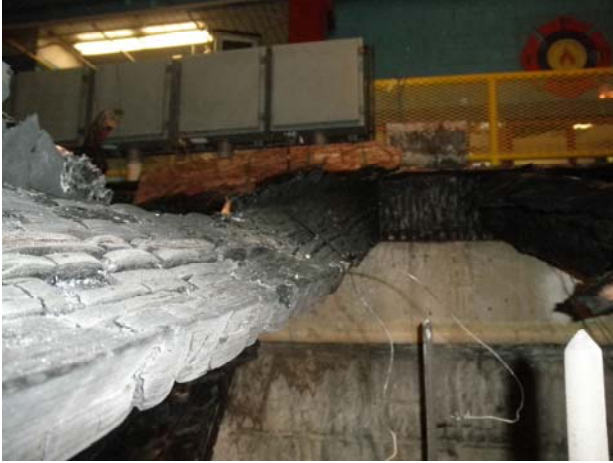
Figure 95. Joist rotation
