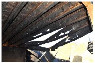
Figure 161 Engineered I-joist at center section of floor area adjacent to rear floor section collapse.
