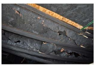
Figure 139 Engineered I-Joist web rupture.
