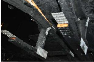
Figure 391 Connection failure of bottom chord tension splice.
