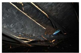
Figure 324 Mechanical separations of the web to flange connections and flange member rupture.
