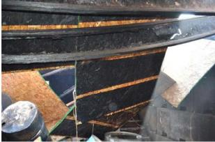
Figure 160 Separation of subfloor due to fastener mechanical separation.
