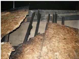
Figure 120 Engineered I-joist web burn-out and sheathing failure at front section of floor system joist bearing.
