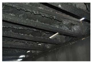
Figure 185 Engineered I-joist web burn-out at bearing condition at front floor section.
