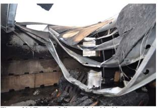
Figure 206 Tearing failure of joist blocking, rupture of lateral bracing strap at underside of floor structure and torsional warping of steel C-joists.
