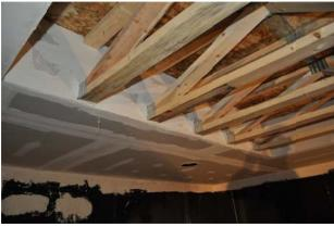
Figure 432. Detailed image showing draft stopping of the exposed trusses
