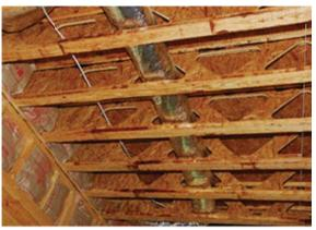
Figure 3. Engineered wood I-beam with cut-outs
