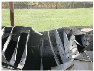
Figure 229. Exterior view of collapsed area of joist bearing condition from above.
