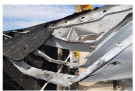
Figure 427. Steel C-joist Loss of strength inducing progressive joist deformations, sheathing connection failure, joist bracing and lateral bracing strap failure
