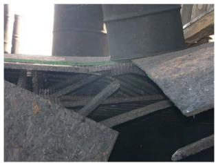
Figure 249 Connection failure at truss panel point.
