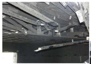
Figure 425. MPCWT Steel to wood panel point connection failure
