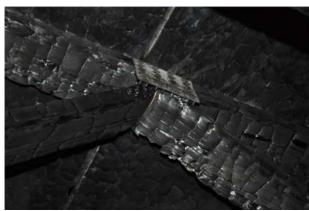
Figure 363 Connection damage at truss panel point.
