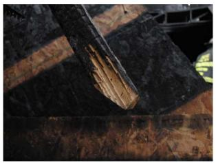
Figure 272 Connection failure at truss panel point.
