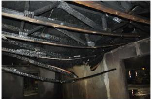
Figure 364 Connection failure of bottom chord tension splice.
