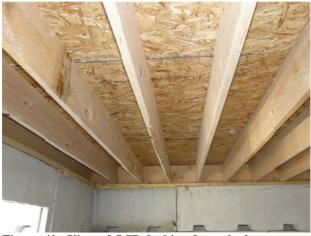
Figure 40. View of OSB decking from the basement
