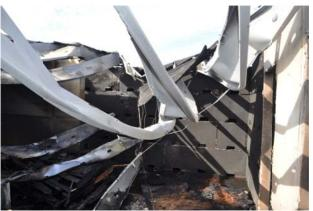
Figure 228 Torsional warping of steel C-joists.
