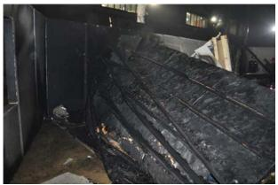
Figure 342 Web burn-out of the engineered I-joist local to collapsed area at front section of the floor system.
