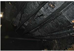
Figure 343 Web burn-out of the engineered I-joist local to collapsed area at front section of the floor system.
