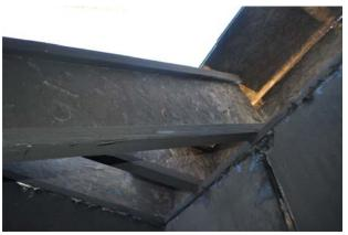
Figure 141 Minimal damage of joist bearing area at front span of floor structure.
