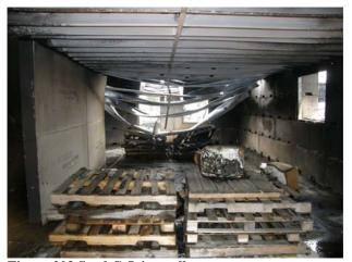
Figure 203 Steel C-Joists collapse.
