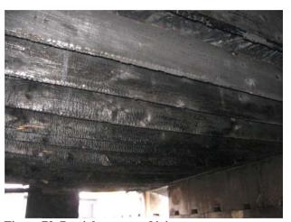
Figure 72 Partial rupture of joists at center span.
