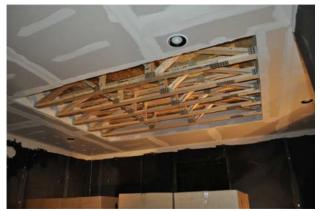
Figure 431. Close view of exposed trusses
