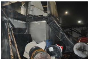
Figure 389 Collapse local to the wood truss bearing condition.
