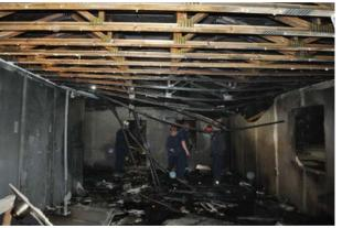
Figure 367 Interior view of condition of floor assembly from underside of floor after remaining drywall removed.
