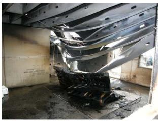
Figure 204 Torsional warping of steel C-joists.
