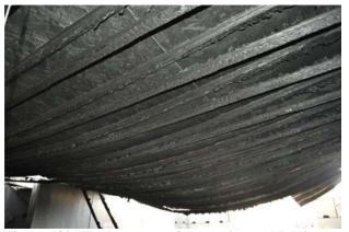
Figure 182 Web burn-out of the engineered I-Joist produced a significant reduction in the joist depth and excessive deflection.
