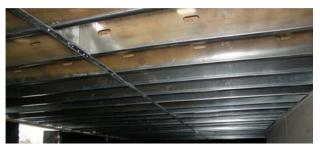
Figure 37. Metal C Joist Floor System
