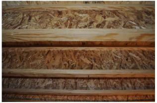
Figure 287. Engineered wood I joists (Exp. A and B)
