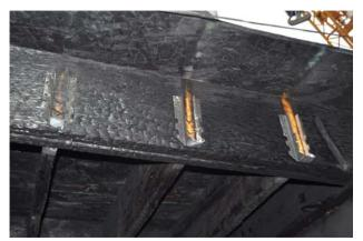
Figure 98 Connections mechanical separation at rear span header support condition.
