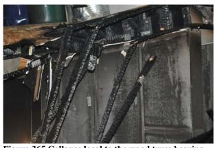
Figure 365 Collapse local to the wood truss bearing condition.
