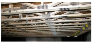
Figure 38. MPCWT Floor System
