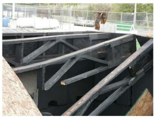
Figure 273 Connection failure at truss panel point.
