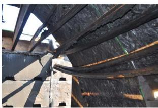
Figure 159 Web burn-out of engineered I-joists at rear section of floor area.
