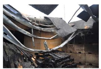
Figure 205 Burn through of sheathing, fastener mechanical separation of sheathing, rupture of lateral bracing strap, and torsional warping of steel C-joists.
