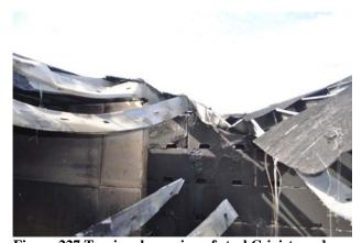
Figure 227 Torsional warping of steel C-joists and collapse local to C-joist support bearing.
