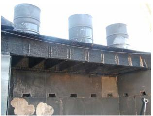
Figure 75 Connection mechanical separation at rear section of floor system header support condition.
