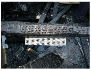
Figure 250 Connection failure at truss panel point.
