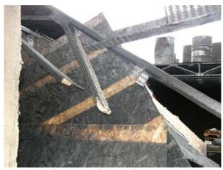
Figure 271 Connection failure of bottom chord tension splice and truss panel point.
