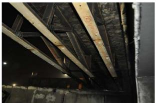
Figure 390 Remaining section of the floor system near the rear of the structure with gypsum board removed
