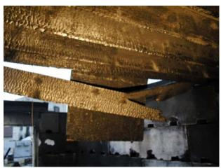
Figure 95 Collapse of ruptured joist at center section of floor system.
