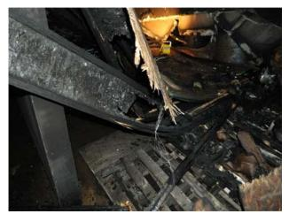
Figure 119 Interior view of collapsed joist at front span.
