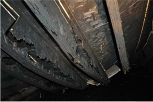
Figure 323 Web burn-out of the engineered I-joist local to collapsed area at center section of the floor system.
