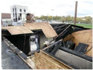
Figure 269 Interior view of percentage of collapsed area from above.
