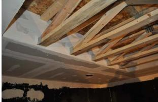
Figure 292. Detailed image showing draft stopping of the exposed trusses
