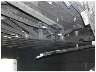
Figure 251 Connection failure at truss panel points and at bottom chord tension splice.
