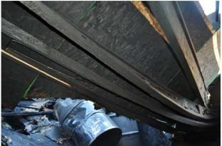
Figure 138 Stability failure of joists, web rupture with separation of sheathing due to fastener mechanical separation.
