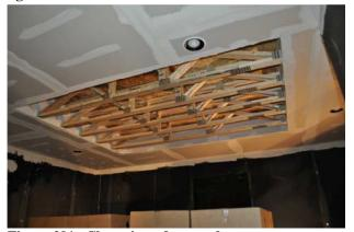
Figure 291. Close view of exposed trusses
