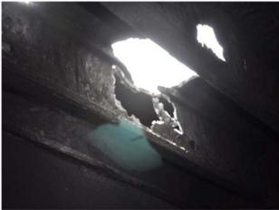
Figure 184 Area of subfloor burn through located at front section of floor system..
