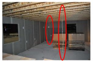
Figure 294. Thermocouple tree locations
