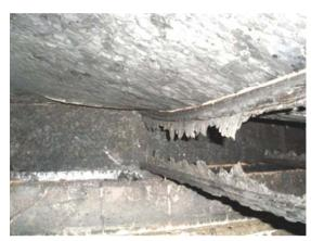
Figure 423. Engineered I-joist Web Burn Through
