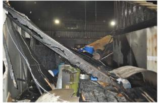
Figure 322 Web burn-out of the engineered I-joist local to collapsed area at center section of the floor system.
