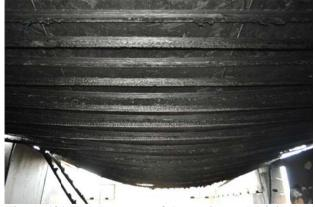
Figure 181 Web burn-out of the engineered I-joist produced a significant reduction in the joist depth and excessive deflection.
