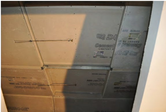
Figure 5.27: Roof Velocity Probes
