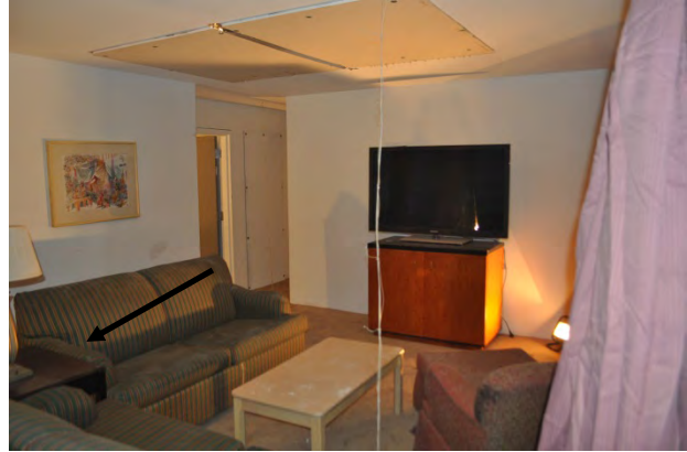
Figure 5.37: One-Story Living Room Ignition Location
