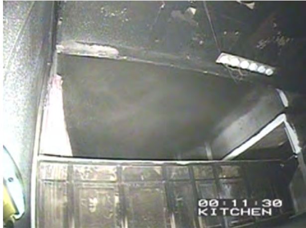
Figure 5.475: Exp. 10 just before roof ventilation looking up to Bedroom fire
