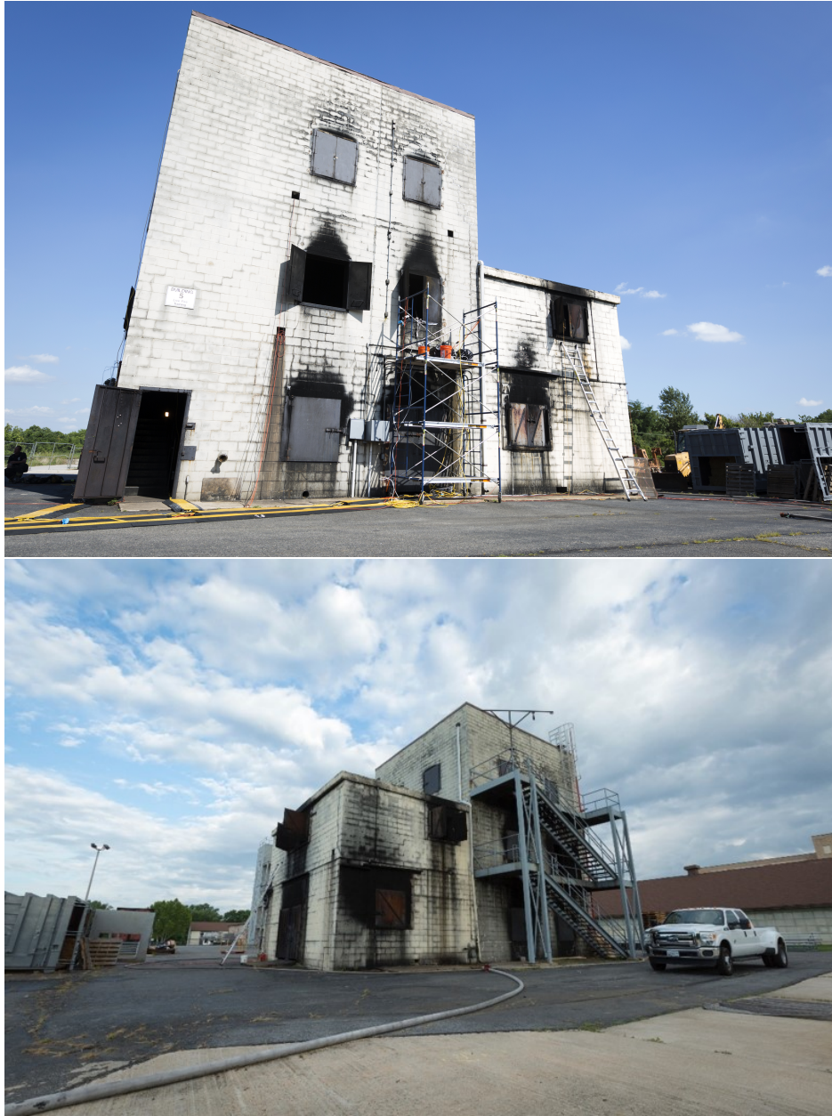
Figure 3.15: Front (top) and rear (bottom) of concrete live fire training building.
